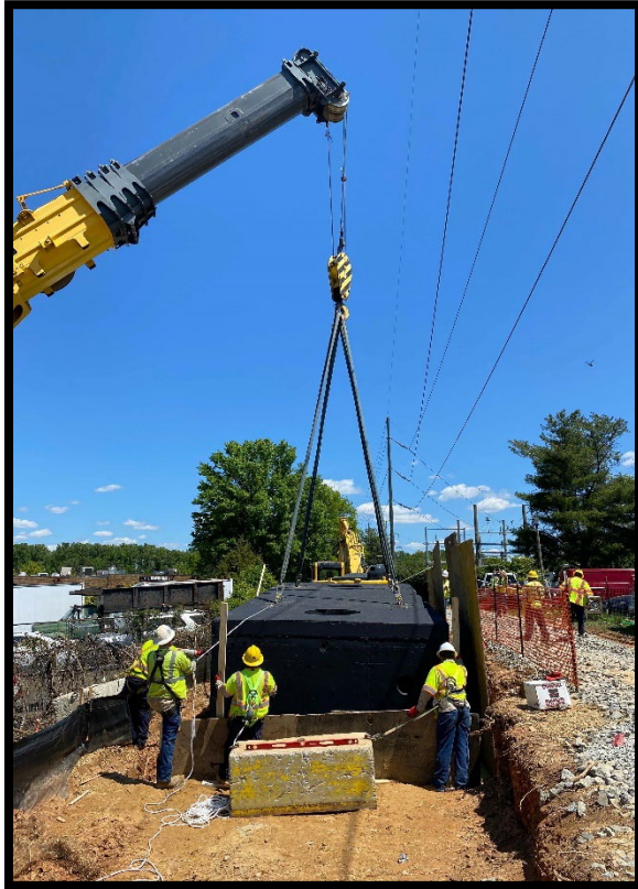
Left Image: Top manhole section being set in place.
