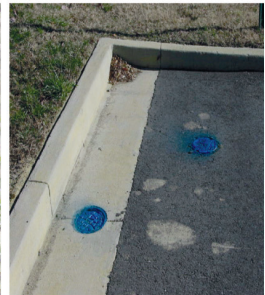
Valve box cover marking
