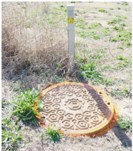
Manhole cover marking
