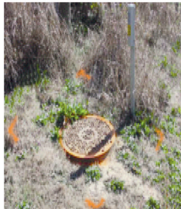
Manhole perimeter marking
