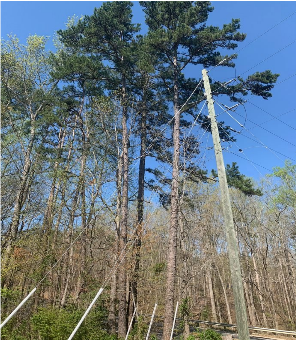
Figure 21. Corner Pole with High Tension
