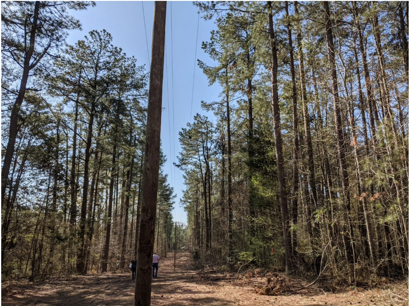
Figure 15. Limbs Overhanging Previously Cleared ROW
