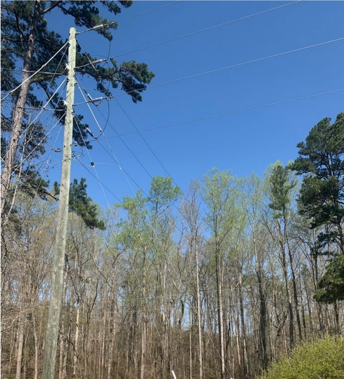
Figure 20. Corner Pole with High Tension
