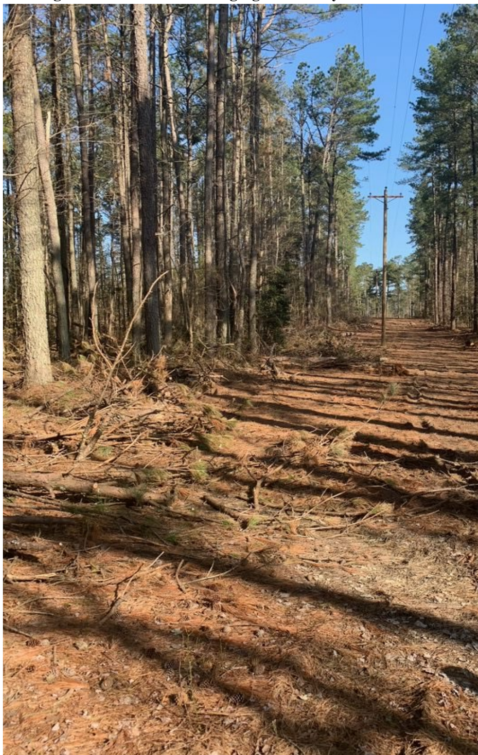
Figure 14. Limbs Overhanging Previously Cleared ROW
