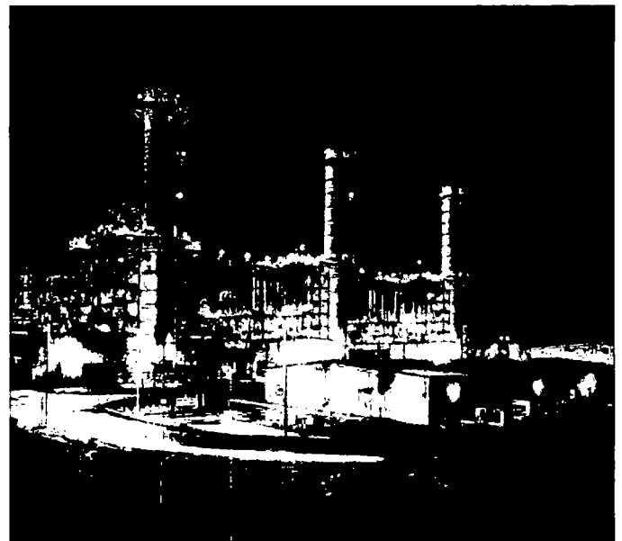
Brunswick Power Station.
