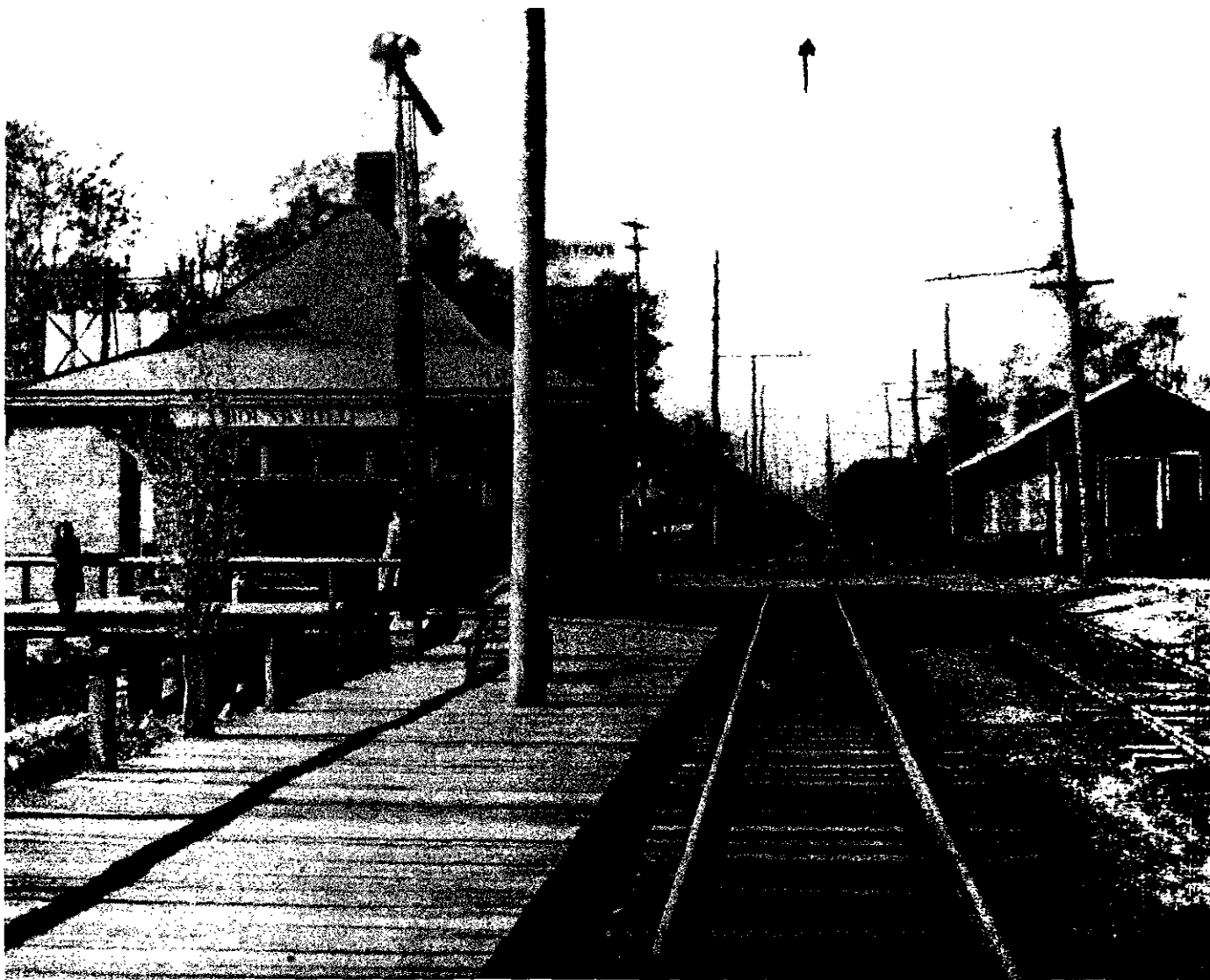
The Southern's Bluemont Branch was electrified using catenary wire suspended from bracket arms on high wooden poles. This early view looks west at Round Hill; the onetime Southern passenger station is at the left with a new electric substation immediately behind it. At the right is the board-and-batten freight house. Both buildings stood in 2000. (LeRoy O. King collection)
