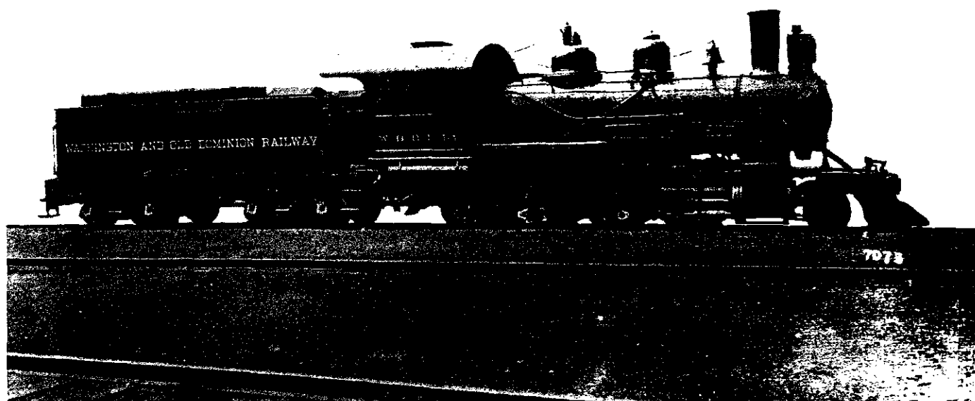
For the W&OD's first 8 years steam power like this shared the tracks with electric cars. The W&OD bought two light 2-8-0s from Baldwin in 1912 for freight and miscellaneous work. Replaced by home-built electric freight motors by 1919, they were resold to the South Georgia Railroad. ( Baldwin Locomotive Works )
