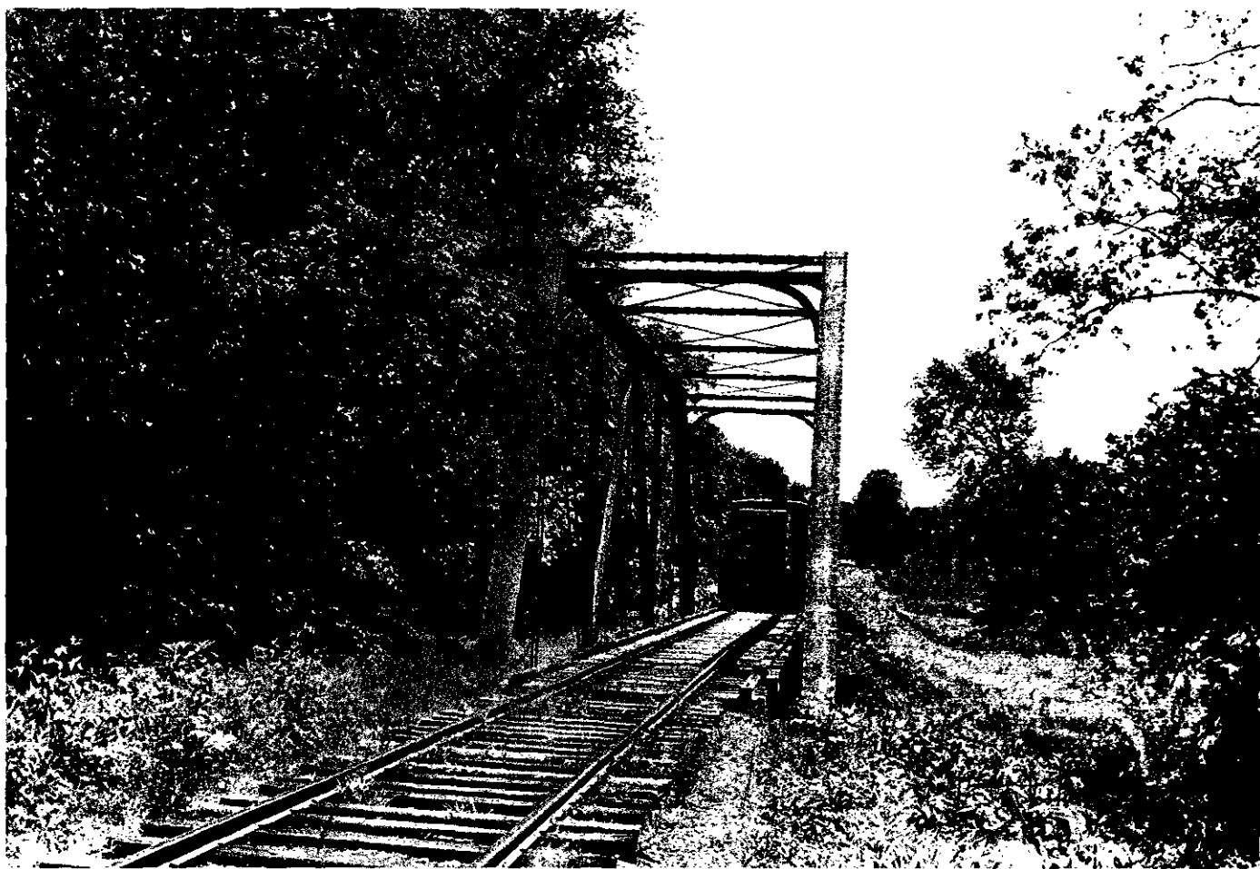
The fragile 1880s-era Difficult Run truss bridge near Hunter's station was an antiquarian's delight and an operating curse. A westbound freight has throttled down to the required 10 mph while its crew hopes for the best. Soon after this 1958 scene it was replaced by a heavy girder span from the C&O. (H. H. Harwood, Jr.)
