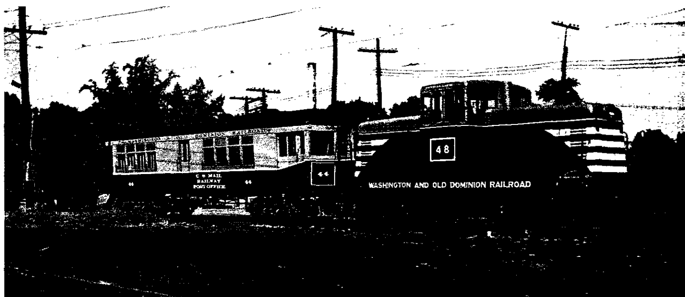
When the wires came down, No. 44 was de-motorized and repainted, and continued its daily mail and express runs behind one of the new GE diesels. Here it readies for its afternoon run at Rosslyn in 1942. Electric wires are still up in the yard. (W&OD)
