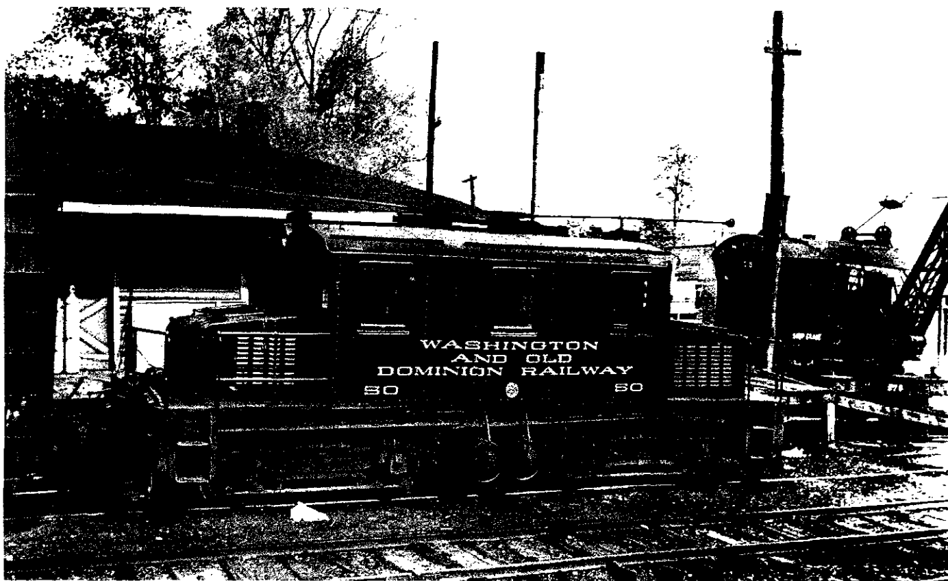
Utilitarian steel freight motors 50 and 51 took over the W&OD's heavier freight chores in the early 1920s. Built to a standardized Baldwin-Westinghouse design, they were rugged and often handled overloads without complaint. Here No. 50 rests in Rosslyn in 1936. As of 1999 it still operated in Iowa—a service life of almost 80 years. (L. W. Rice)
