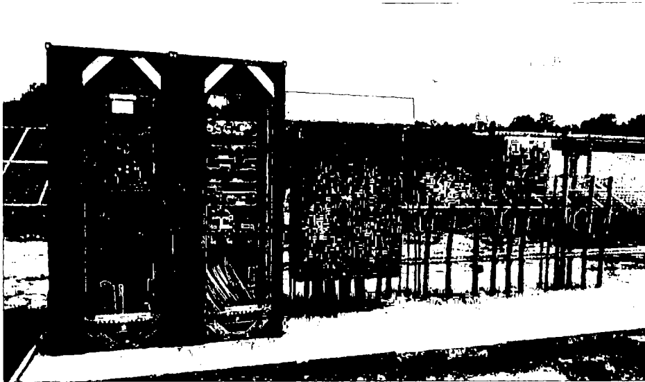
Exhibit 9: Merck solar project main switch gear and interconnection metering equipment
